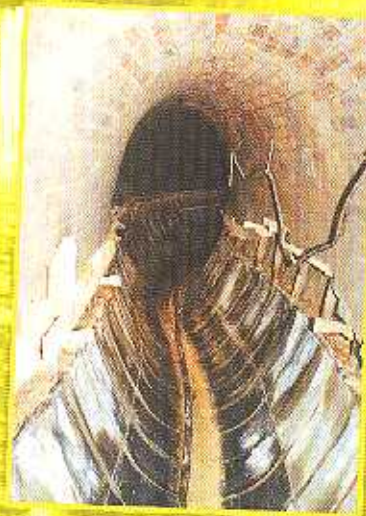
Reconstruction of underground sewage conduit in Prague. Cast Basalt troughs and side plates are applicated.
