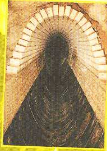
Reconstruction of underground sewage conduit in Prague. Cast Basalt troughs and side plates are applicated.
